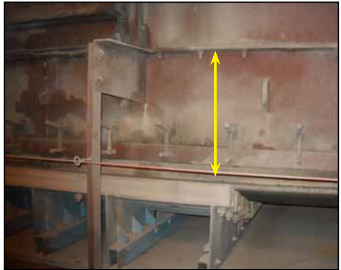
Conveyor surface to top of skirt board
