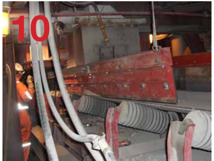
Lifting a 15-foot (3-doors) assembly into place.
