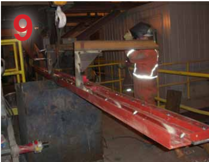
Attaching Support Structure every 5-feet.
