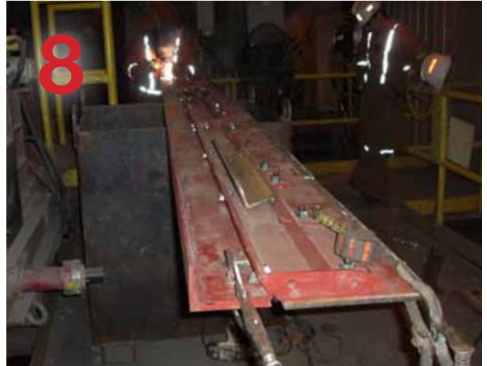
Attaching 15-foot long 3 x 5 upper support angle.
