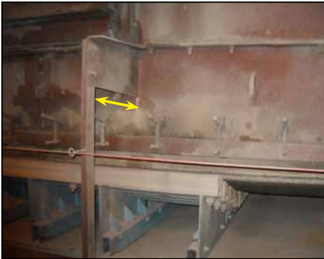
Inside of vertical support to skirt board
