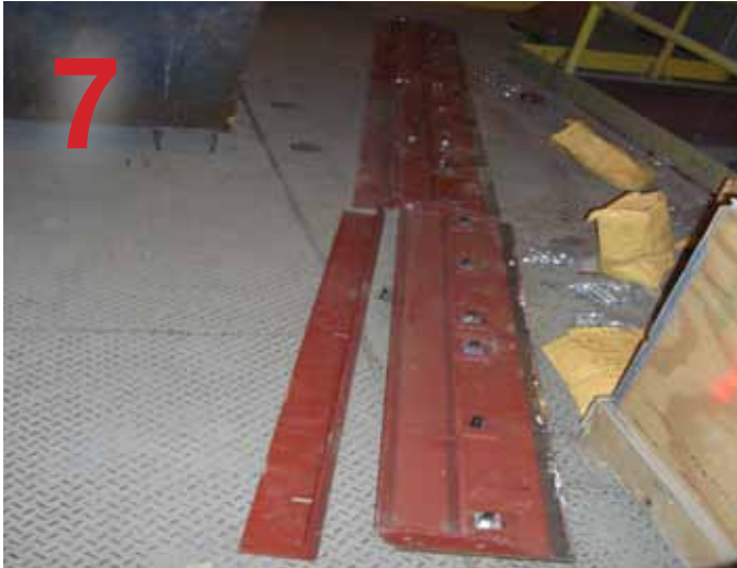
Three EZ-ACCESS™ Assemblies being attached end to end. Upper flanges being attached also.
