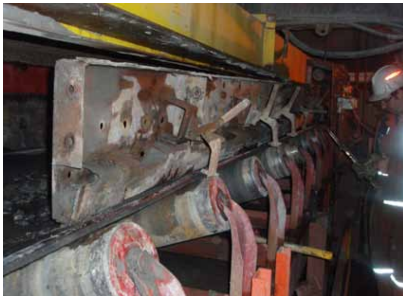
Removing old skirt board
